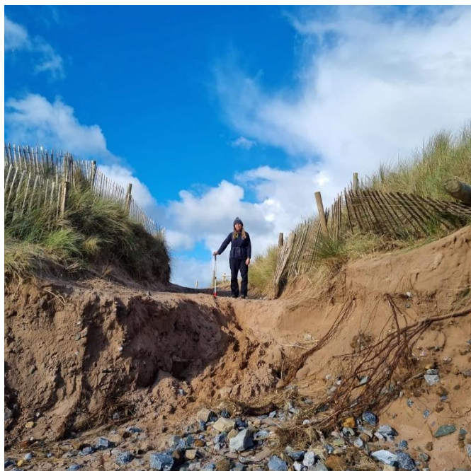
Figure 7. Storm damage/erosion at Dawlish Warren NNR.
